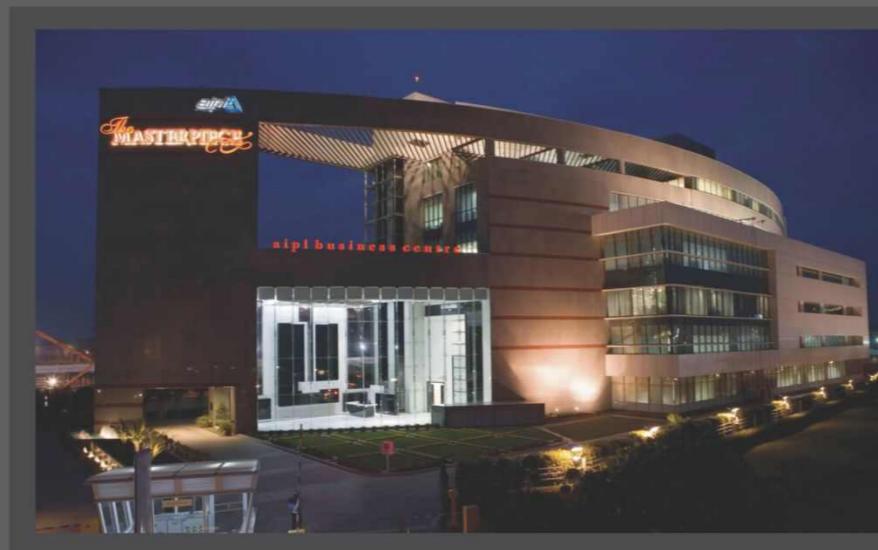
The Masterpiece, Golf Course Road, Gurgaon
