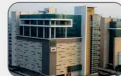
GREENFORT, NOIDA India's Finest Data Centre For City
